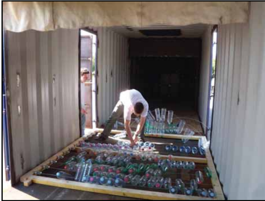
Figure 17. “Bottle frame” construction, inside the compartment
